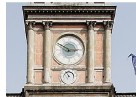
Clock with auxiliary dial displaying the equation of time. Piazza Dante, Naples (1853).
